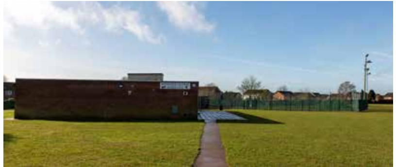
The new MUGA would be installed at St David's recreation ground. Photo by Ian Topham
